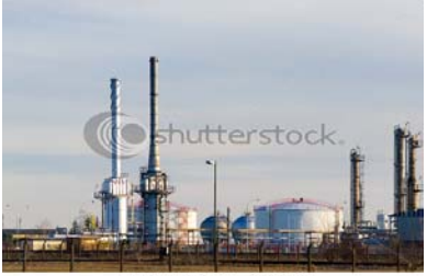
Natural Gas Refinery
